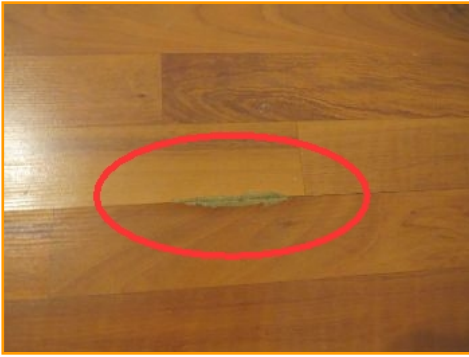
Moisture Damaged
