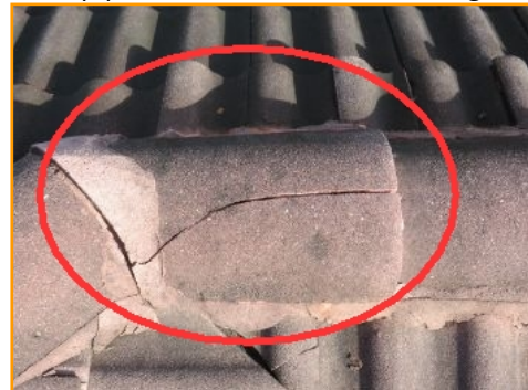
Damaged/Cracked Roof Tile(s)
