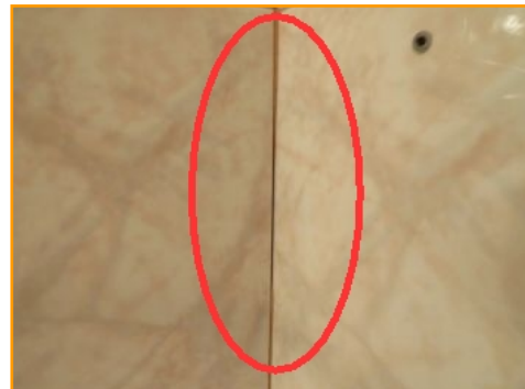
Deteriorated Grout
