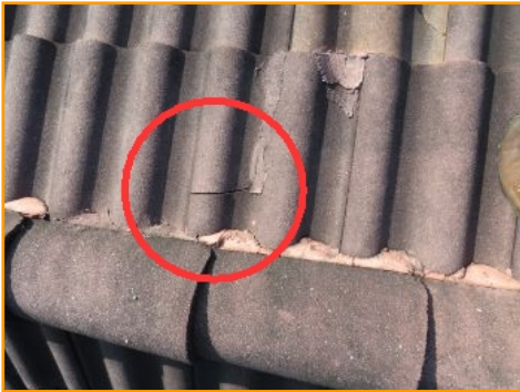
Damaged/Cracked Roof Tile(s)
