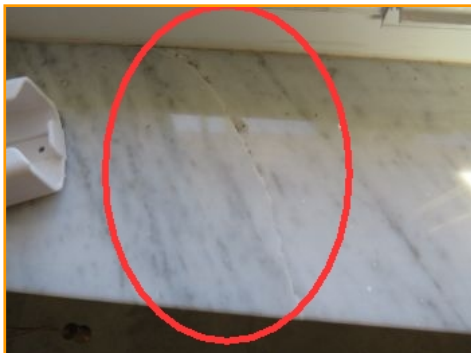
Damaged Window Sill
