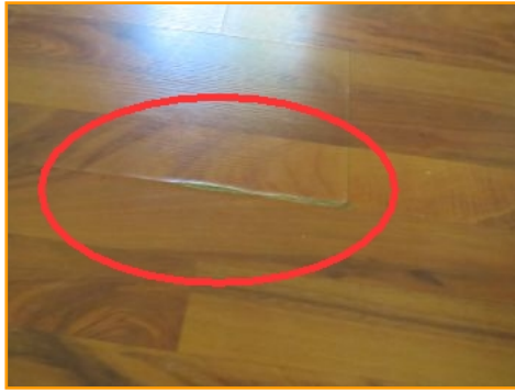
Moisture Damaged
