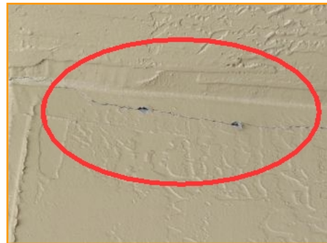
Stucco Damage/Cracks
