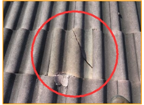
Damaged/Cracked Roof Tile(s)
