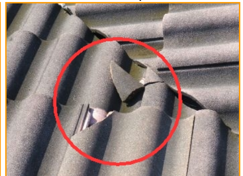
Damaged/Cracked Roof Tile(s)
