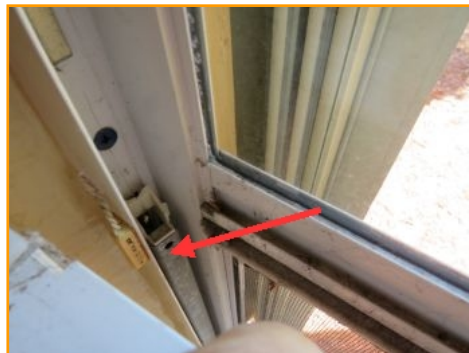
Damaged Springs/Tension Rods
