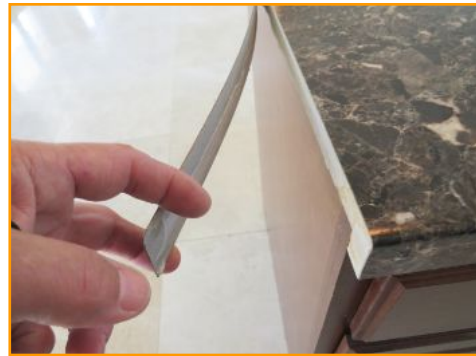
Loose/Damaged Laminate
