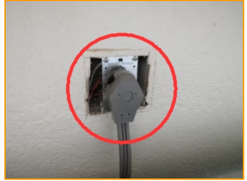
Missing Face Plate/Cover
