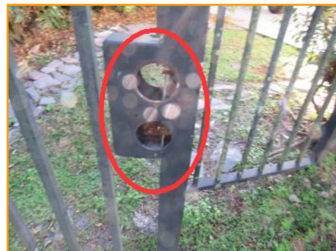
Damaged/Missing Hardware
