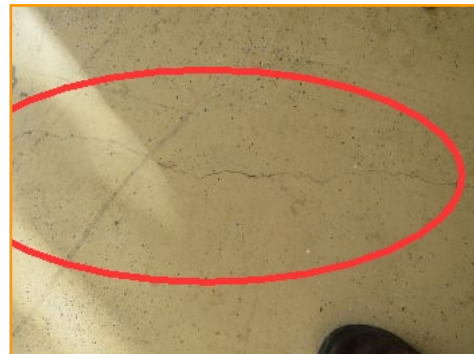
Settlement Cracks
