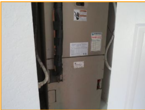
AC (Cooling/Heating) Air Handler #3
