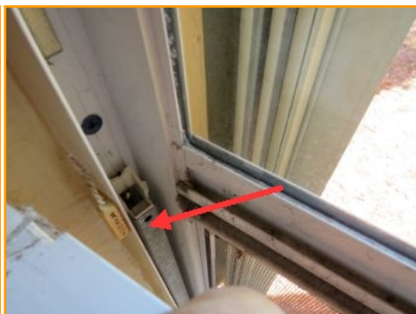
Damaged Springs/Tension Rods Damaged Springs/Tension Rods Damaged Springs/Tension Rods
