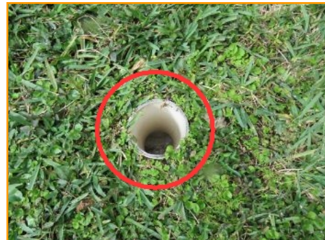
Clean Out Cover's Missing
