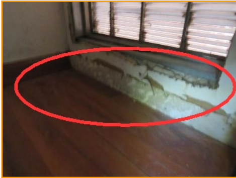
Moisture Damaged
