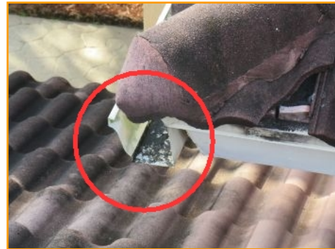
Draining Onto Roof
