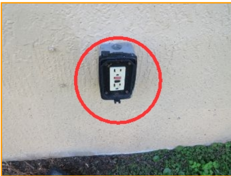
Missing/Damaged Weather Cover
