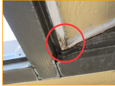
Moisture Damaged Fascia
