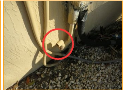
Condensate Near Foundation
