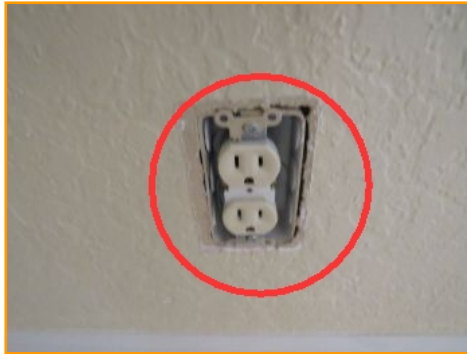
Missing Face Plate/Cover
