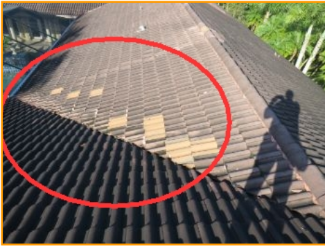
Previous Roof Repairs
