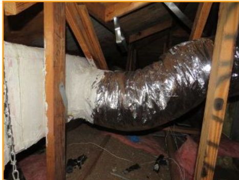
AC (Cooling/Heating) Ductwork
