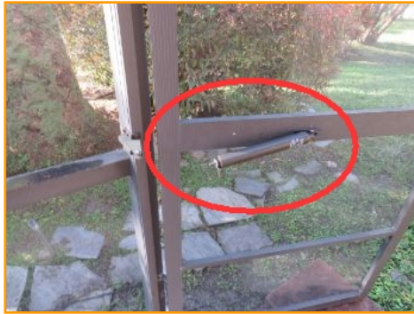
Damaged Door Strut
