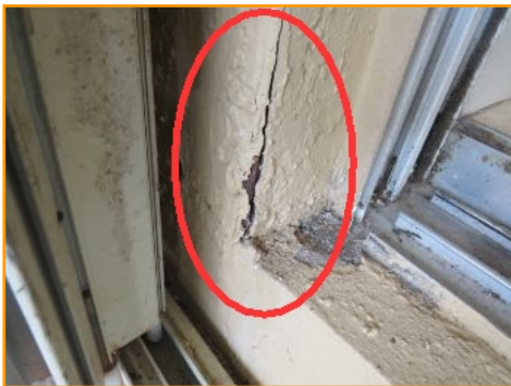
Stucco Damage/Cracks
