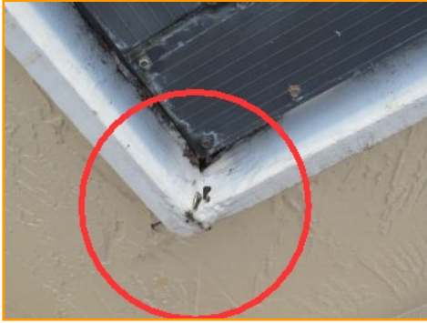
Moisture Damaged Fascia
