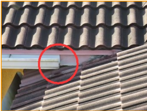
Draining Onto Roof
