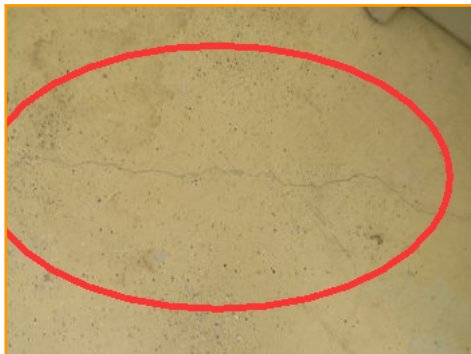
Settlement Cracks
