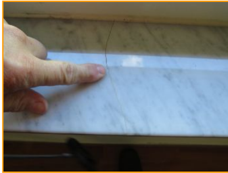
Damaged Window Sill
